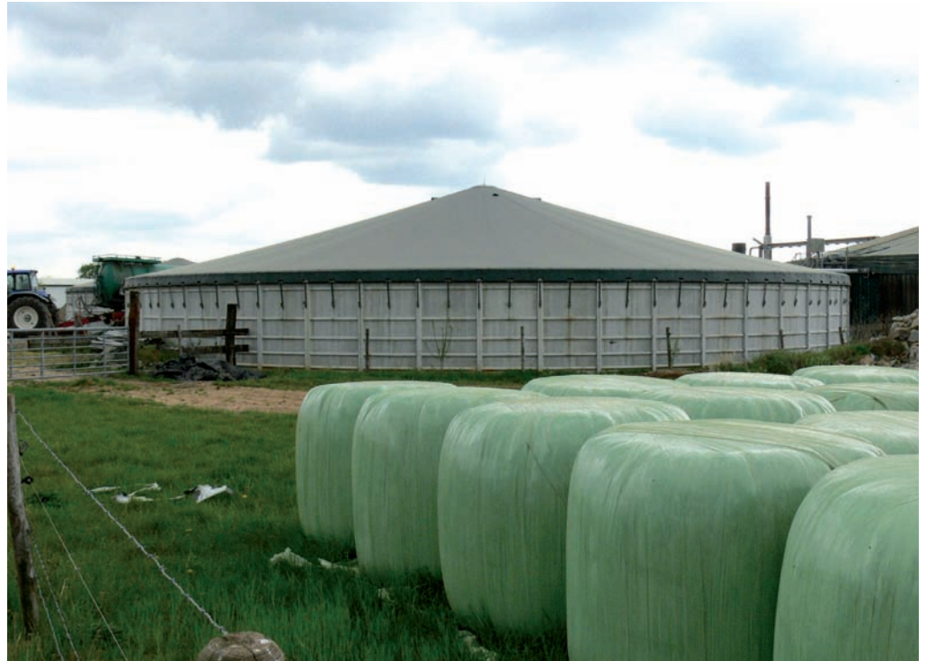
The biomass installation which heats Georg Welzel's greenhouses.
